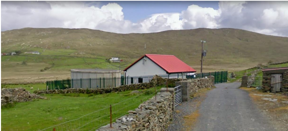
The Treatment Plant for lough Cumnel Group Water Scheme ( Google Earth )
